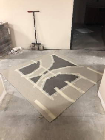
These photos highlight the flooring and finish millwork below. The main flooring has been installed and the logo details are in progress.
