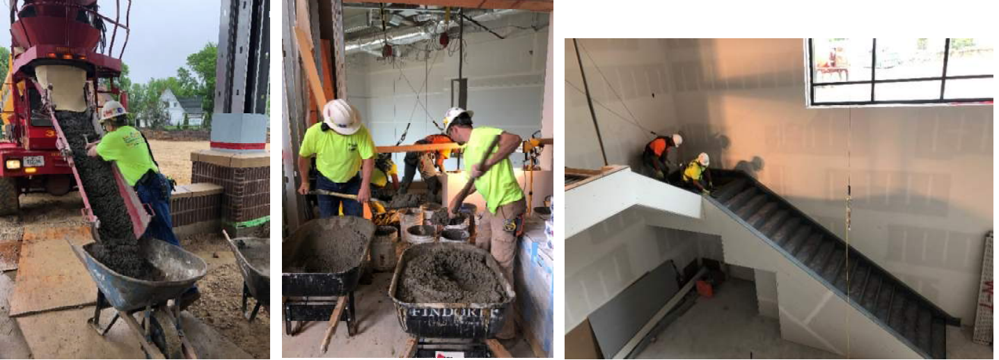
The photos above depict the various steps required in order to install the concrete on the Grand Stair. Wheel barrels are used to haul the concrete from the pump truck into the building and then shoveled into buckets to be carried to each step and poured into place.
