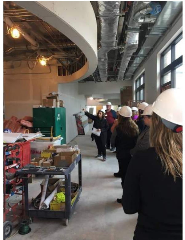
An owner representative led tour through the Main Street area in the upper level to show the hospital employees the construction progress.
