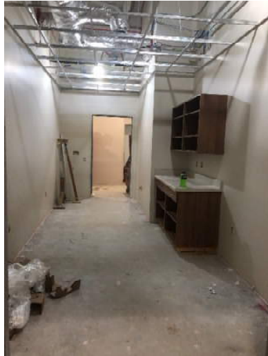
In the upper level Med Surge / Clinic addition, bathroom tile is being installed as well as millwork and the ceiling grid. After these go in, the MEP trades will go through and install their fixtures such as sinks and lights.
