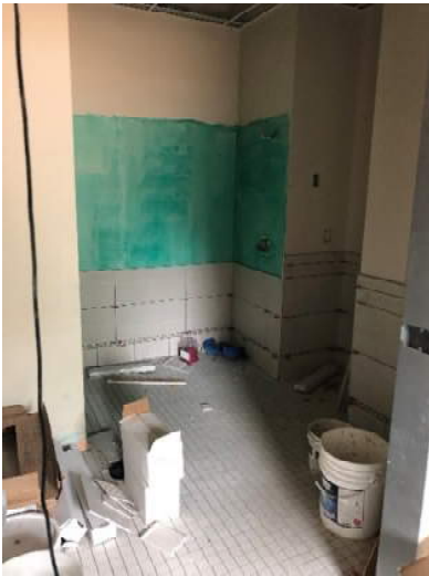
In the upper level Med Surge / Clinic addition, bathroom tile is being installed as well as millwork and the ceiling grid. After these go in, the MEP trades will go through and install their fixtures such as sinks and lights.
