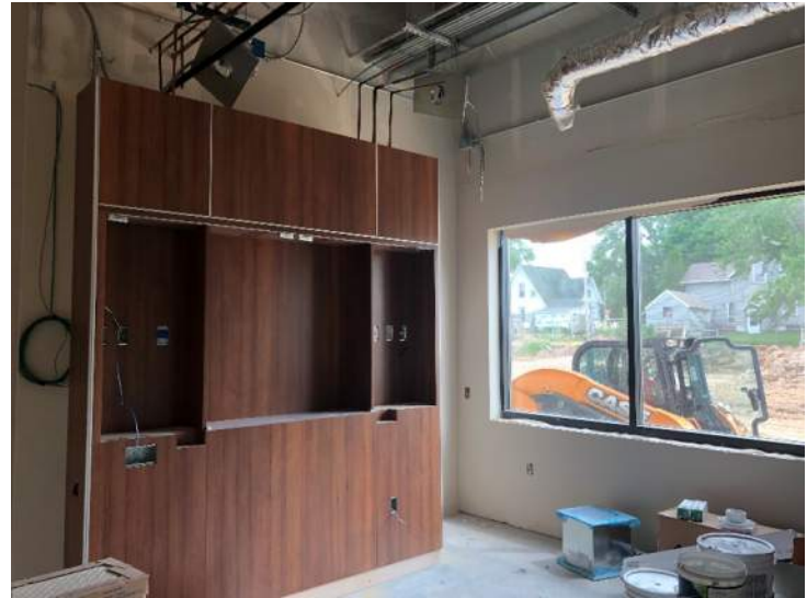
A headwall unit is placed in its final resting location after the MEP rough ins have been installed. The next step will be to install the MEP trim within the unit.
