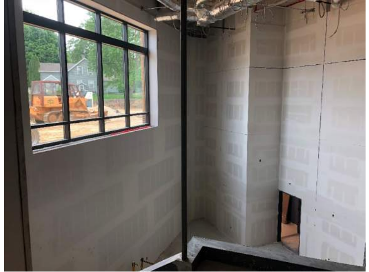
A view from the top of the Grand Stair peering down into the registration area of the lower level Med Surge / Clinic addition.
